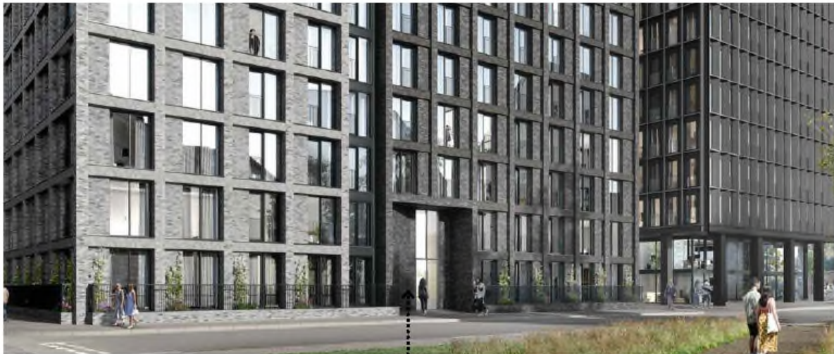
Hulme Hall Road Elevation
