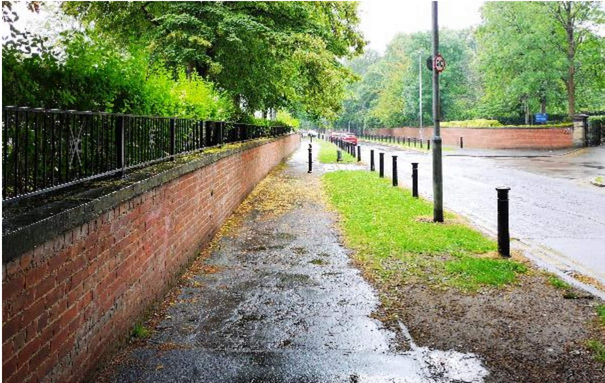
View looking southwards along Lower Park Road, the boundary wall and railings to Ward Hall is on the left of the picture
