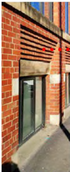
Brick detailing to openings - Britannia Mill
