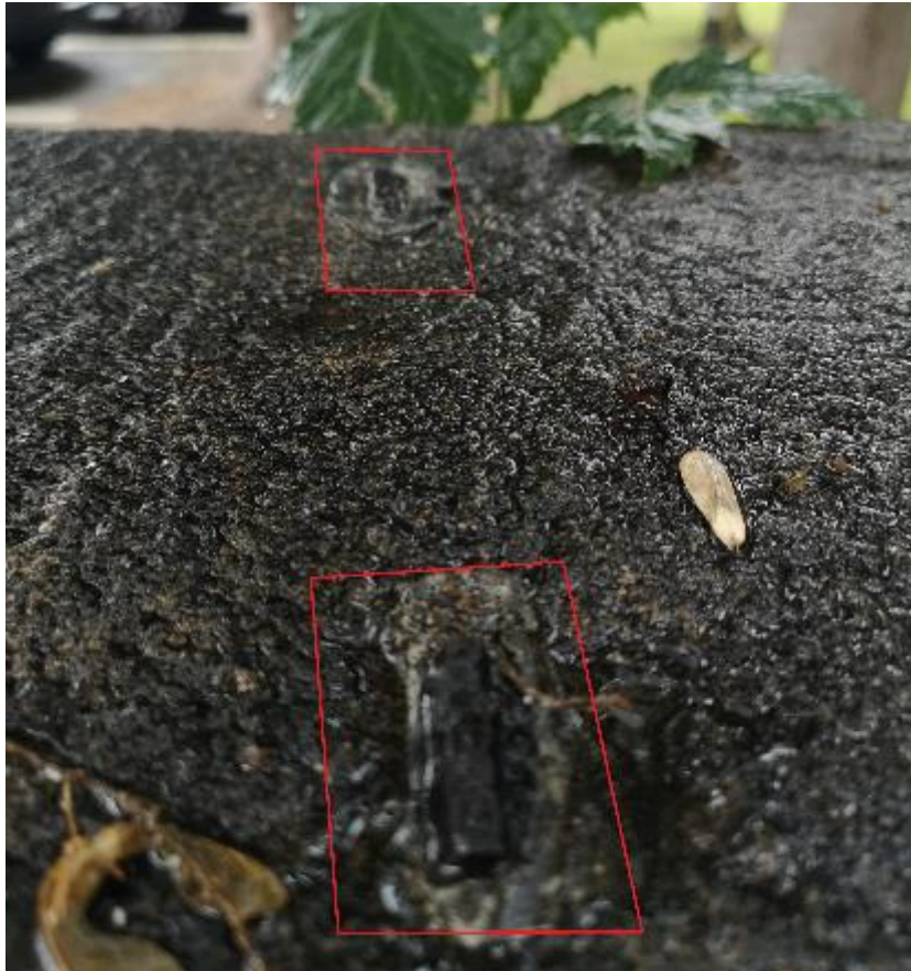
Remnants of former railings on boundary wall at Xaverian Campus
