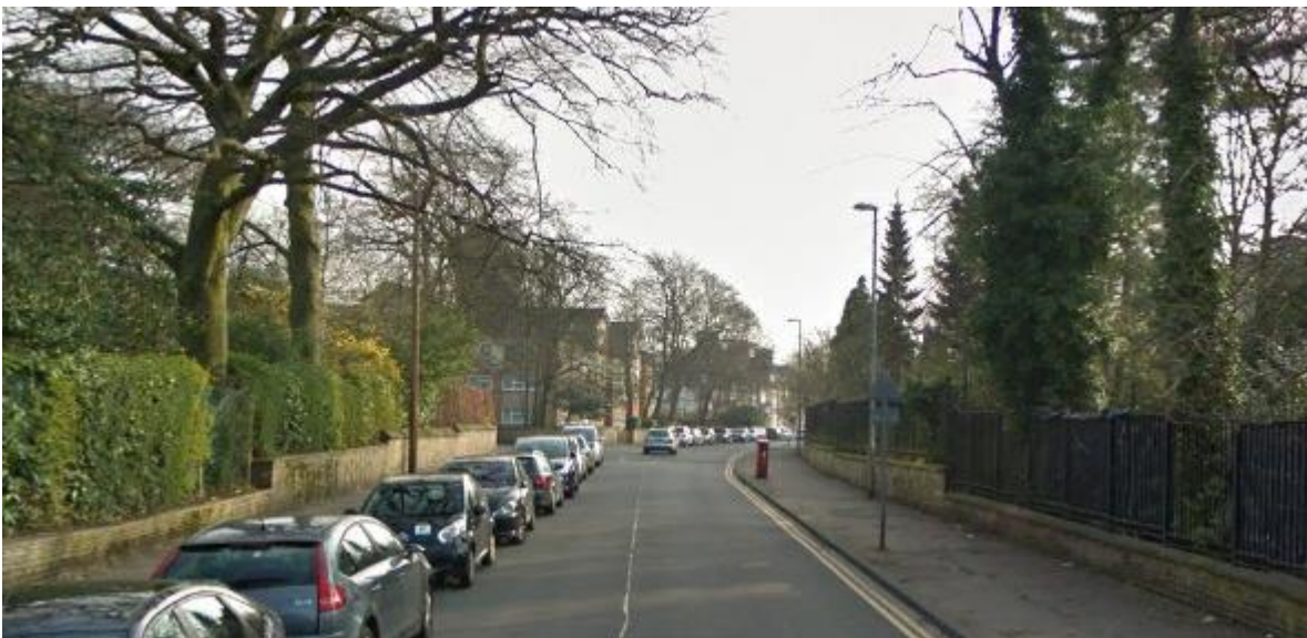
Denison Road looking east – Low stone walls with railings(right), low wall with hedging (left)
