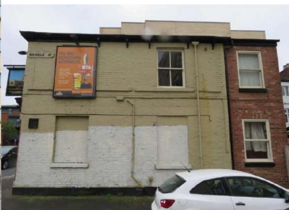
(Side Elevation from Brindle Street)
