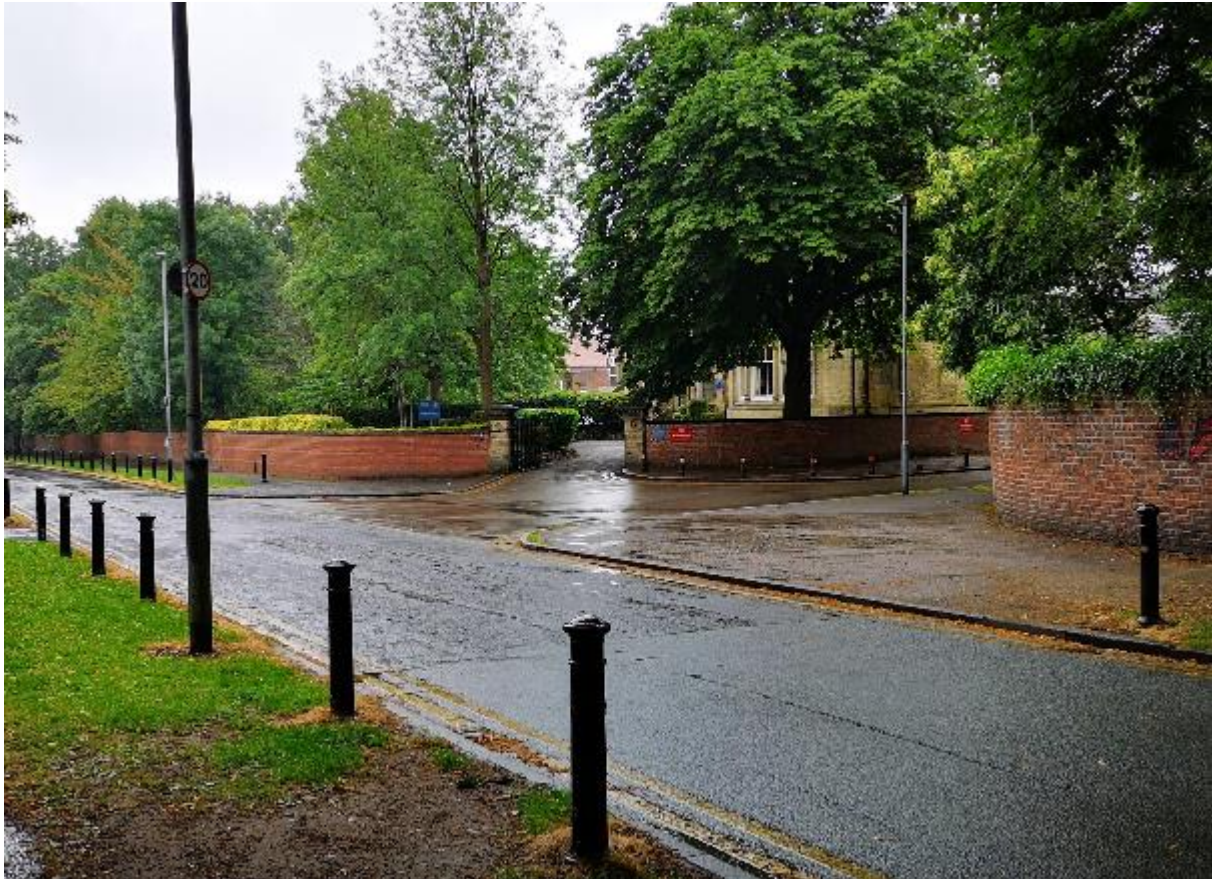
Entrance gates and posts and boundary walls to the front of Marylands
